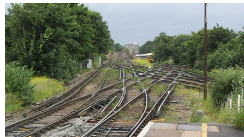
The flat junction at Lewisham station prevents effective peak operations.
